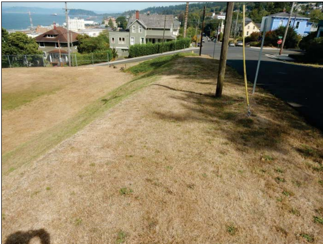
Figure 7: View east along Grand Avenue near the top of the proposed children's slide. The groomed slope on the left drops at about 50 percent and appears to be reasonably free of hummocks or indicators of slope instability, except for the slope where the shadow of the telephone pole falls, where it appears to bulge out on the slope and to have settled on the grassy shoulder. This possible instability lies east of the preferred construction site.
